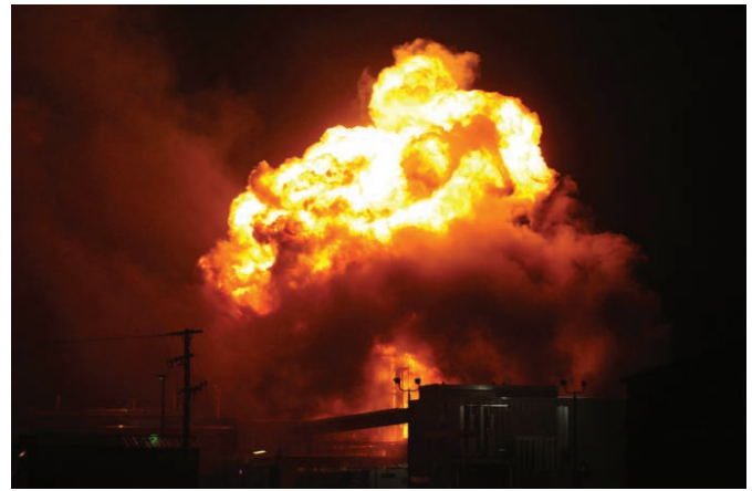
Ohio oil refinery explosion 2015
