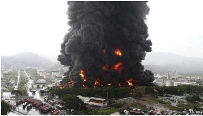
Venezuela Puerto La Cruz refinery fire 2013
